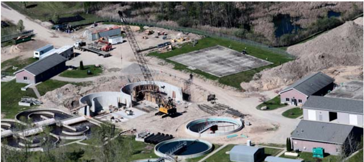
The wastewater treatment plant under construction (2015), a planned upgrade to increase the capacity from 1.2 to 2.4 MDG.
