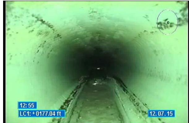
Sample shot from televised inspection – within gravity sewer between MH#227B & MH#227A on River Road
