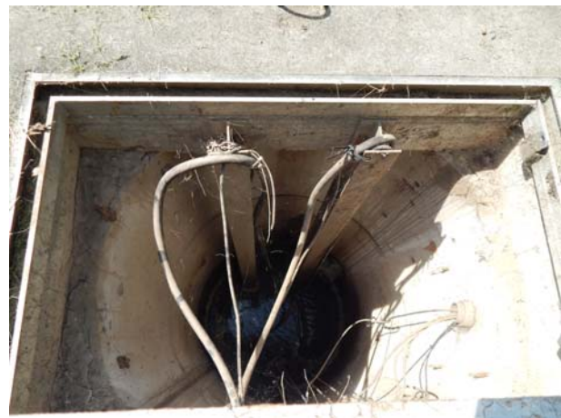
Pump Station #8 (Scully Drive)
