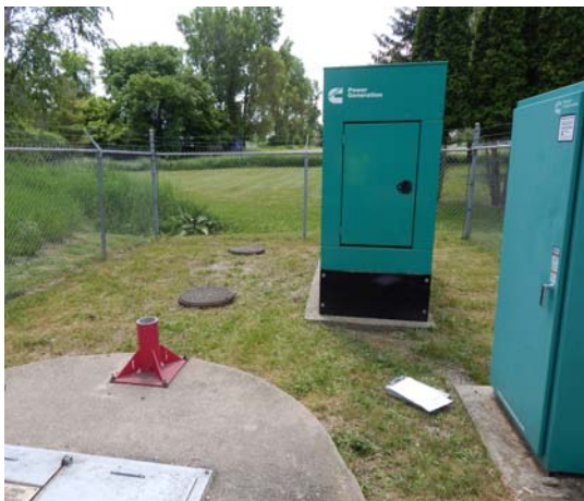
Pump Station #7 (McDonald Drive)
